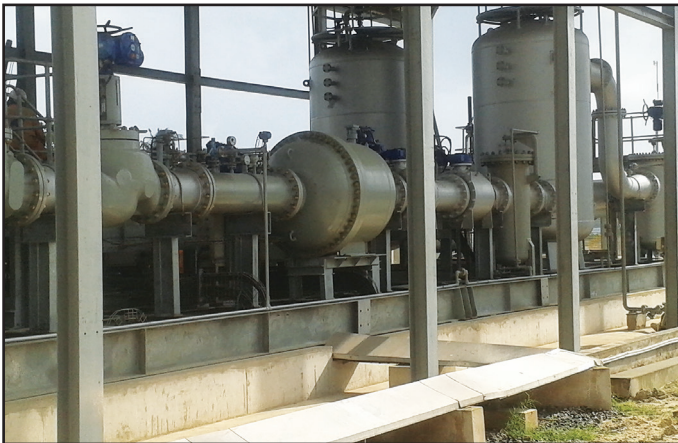
Dual 16" Line Metering Skid
