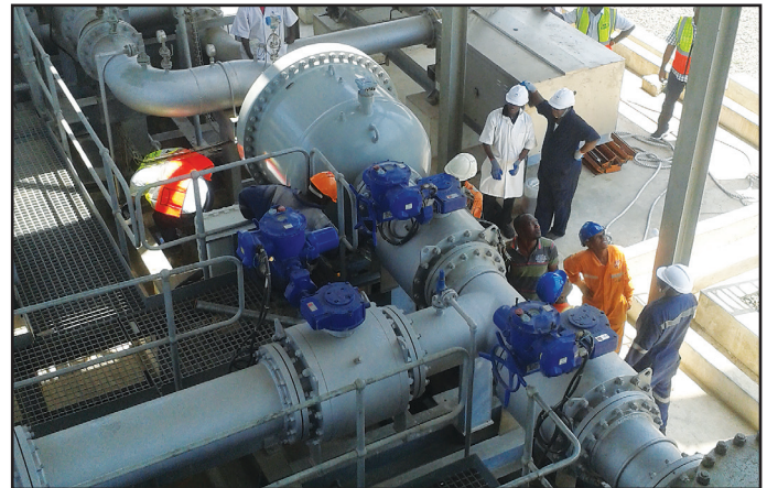
Dual 16" Line Metering Skid
